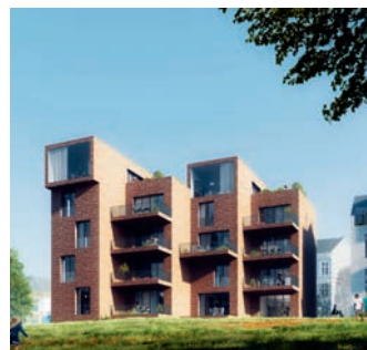
Oslo gate 7, Oslo
